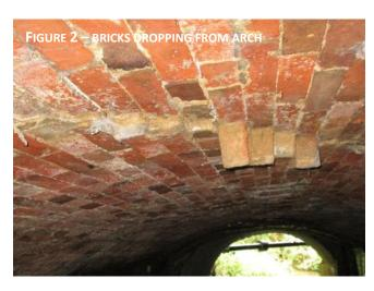
Due to the volume of traffic and number of heavy vehicles using the route, Northamptonshire Highways took the operational decision to close the A422, to allow temporary propping to be installed before the arch collapses, and allow the road to be reopened, probably under signal control. This will be carried out as quickly as possible, once the temporary props are designed.
